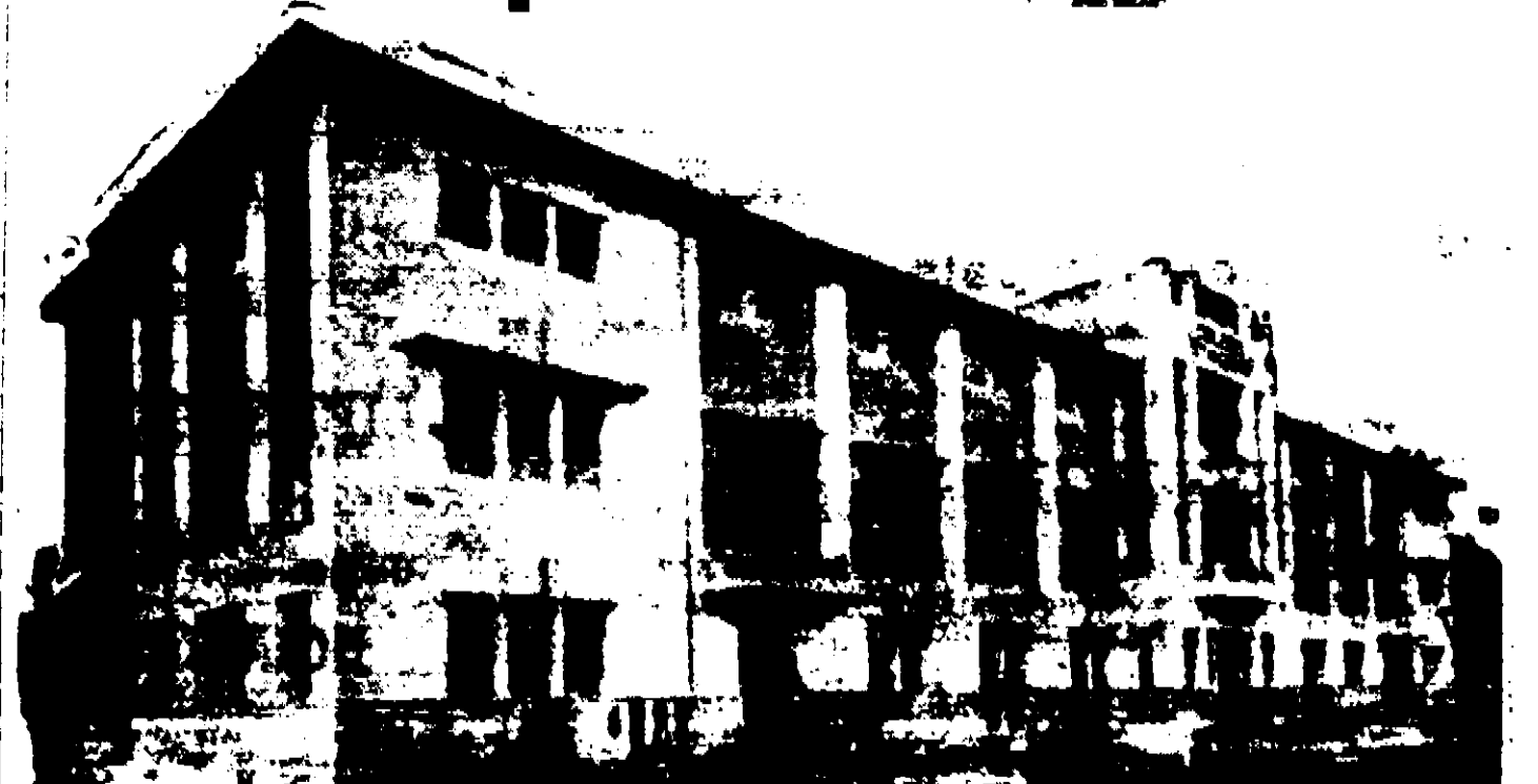
Fachada principal do Colegio Santo Antonio
