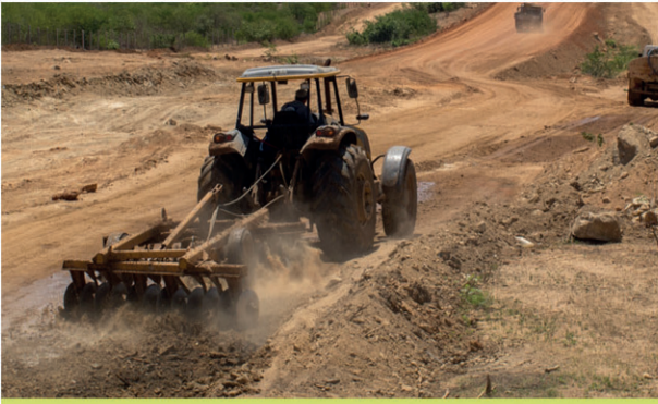
RETOMADAS AS OBRAS NA BR-226
