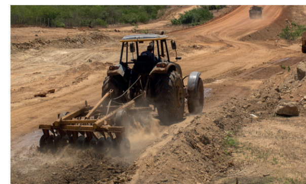
RETOMADAS AS OBRAS NA BR-226
